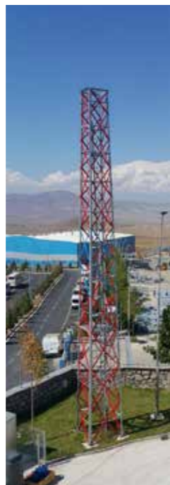
A Hybrid Composite Tower Application: Blue and red profiles are FRP.
