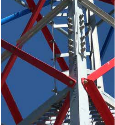
A Hybrid Composite Tower Application: Blue and red profiles are FRP.
